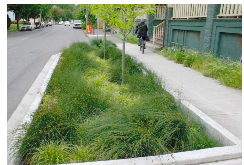
Chicanes designed to double as rain gardens
