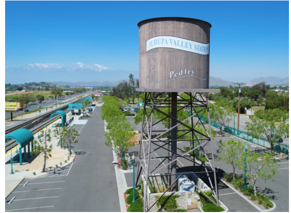
Pedley Station provides regional transportation via Metrolink and Riverside Transit Agency bus transit.
