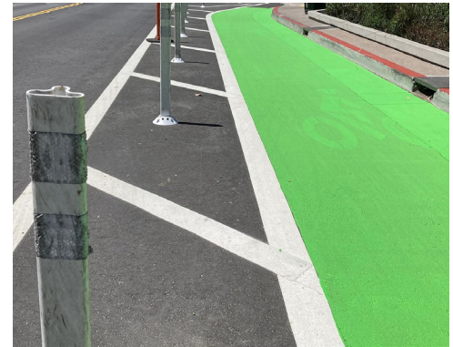
Striped buffers with flexible / reflective bollards for additional visibility.
