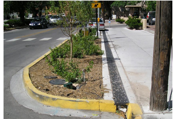
A mid-block bulb-out protecting a pedestrian crossing with existing street gutter maintained.
