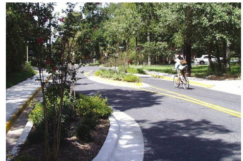
Example of Class III Bike Route on a neighborhood street with additional traffic calming features (chicanes & medianettes)
