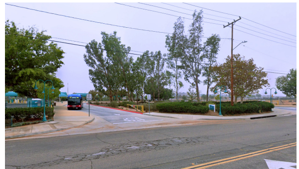
Existing RTA bus depot at north end of Pedley Station
