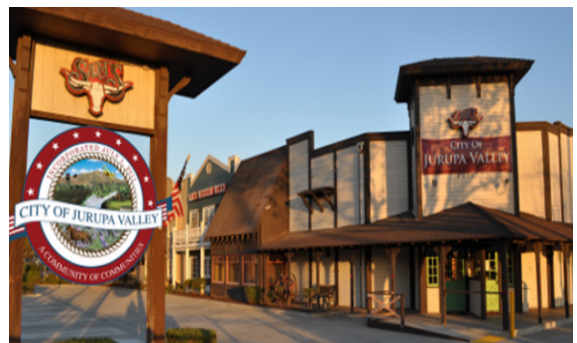
Plans are currently underway for the expansion of City Hall, with the potential for it to become a prominent anchor to a growing civic center district in Pedley.
