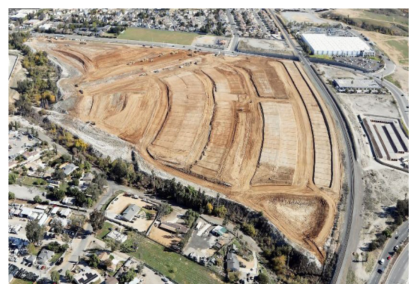
Rock Rose & Bayberry Pointe, currently under construction will add another 254 single-family homes to Pedley.
