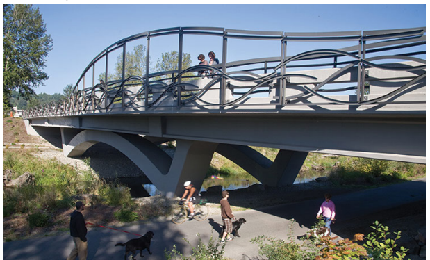
A pedestrian overpass can be functional and sculptural, becoming a local landmark that draws visitors from around the region.
