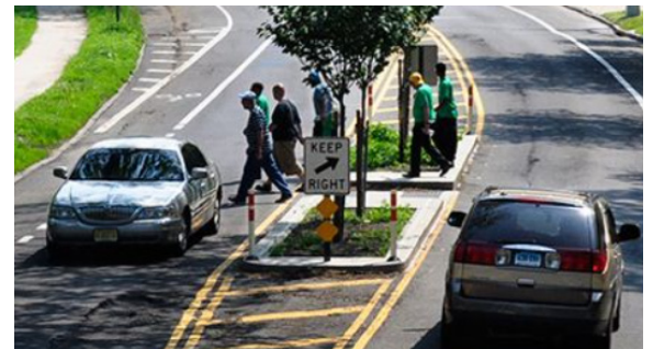
Mid-block crossing with a medianette pedestrian refuge
