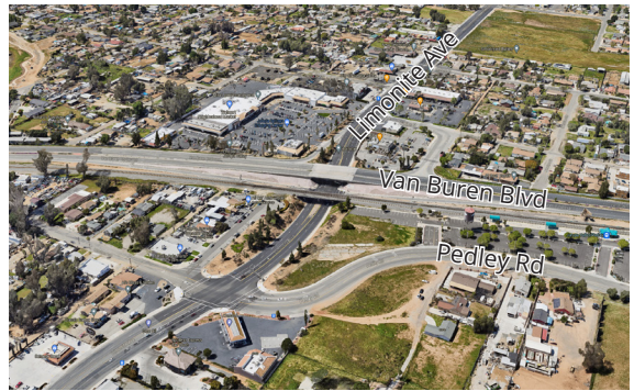
Van Buren Boulevard is a significant physical barrier, effectively bisecting the Pedley Town Center area into “East” and “West” quadrants.
