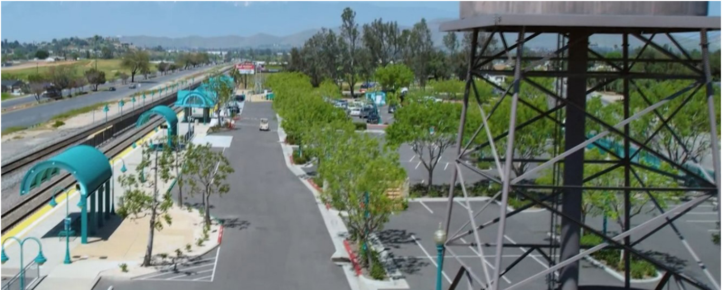
The Metrolink Station area
