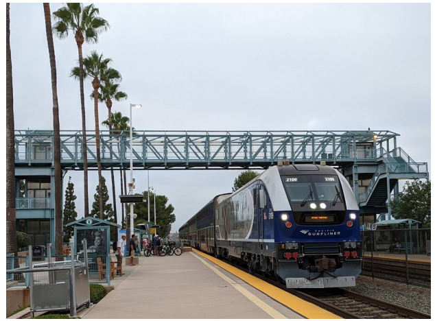
Pedestrian/Bicycle rail overpass
