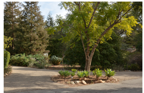
Neighborhood traffic circles need not be circular. This triangular-shaped planted area slows down traffic while beautifying the street.
