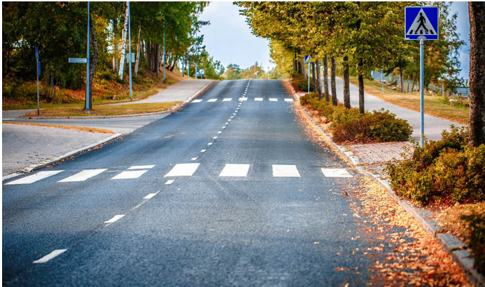
Even rural crosswalks should be clearly marked with painted stripes and signage
