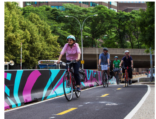
Physically separated bike lane going through an underpass
