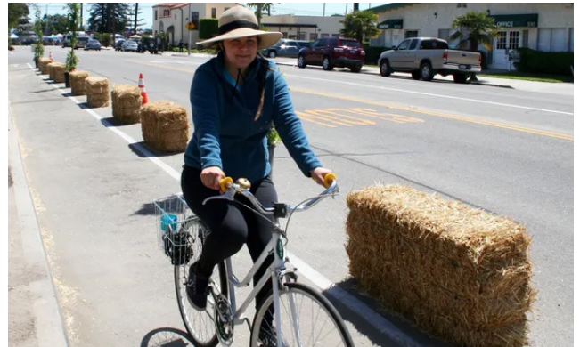
Example of tactical impementation / testing of a protected Class IV bike lane - using hay bales - on an arterial corridor in Oxnard, CA.
